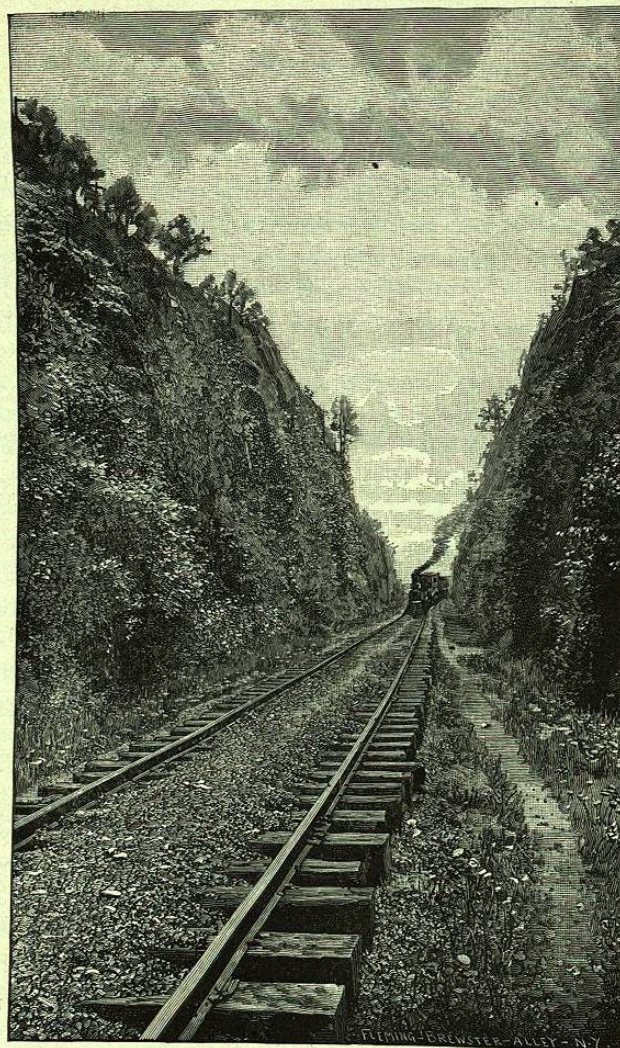
RAILROAD CUT, ALLATOONA. FORT "C" ON THE LEFT, FORT "T" ON THE RIGHT.
