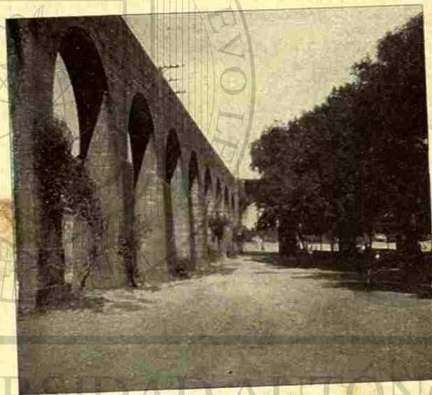
THE AQUEDUCT, MORELIA.
