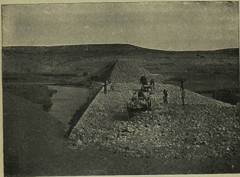
FIG. 33.—LAKE AVALON DAM. ROCK-FILL IN PROCESS OF CONSTRUCTION.
