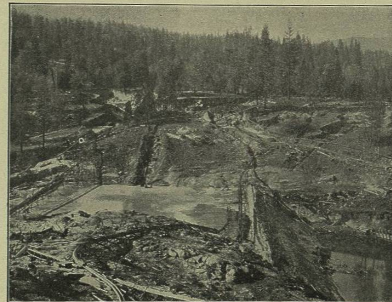
FIG. 82.—BORROW-PITS FROM WHICH MATERIAL WAS SLUICED TO THE CRANE VALLEY DAM IN BACKGROUND.
