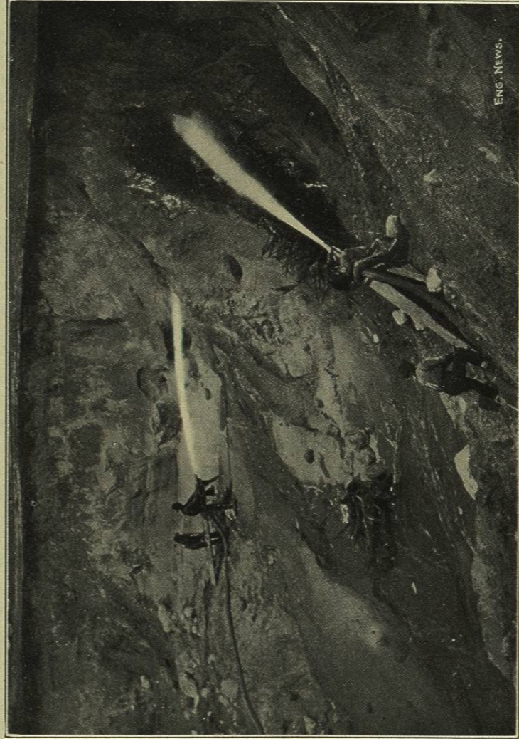
FIG. 139.—HYDRAULIC SLUICING ON THE CROTON DAM, SHOWING THE IMPROVISED NOZZLE CONTROL, OR HYDRAULIC MONITOR. 181
