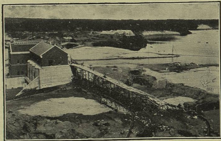
FIG. 137.—CROTON HYDRAULIC-FILL DAM, MICHIGAN, DURING CONSTRUCTION.
