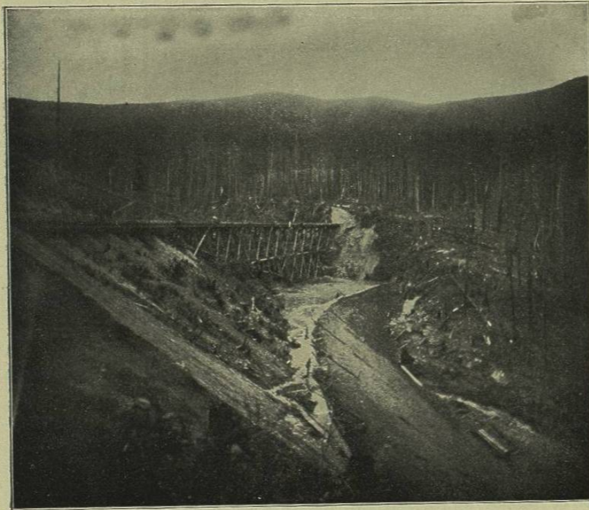
FIG. 146.—NORTHERN PACIFIC RAILWAY, BRIDGE 184. HYDRAULIC FILLING IN PROGRESS.
