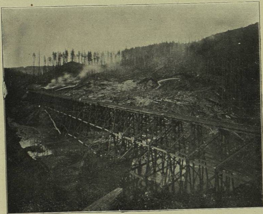
FIG. 144.—NORTHERN PACIFIC RAILWAY. BRIDGE 189, CASCADE MOUNTAINS.
