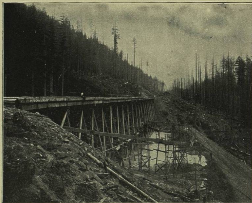
FIG. 143.—NORTHERN PACIFIC RAILWAY. BRIDGE 190.
