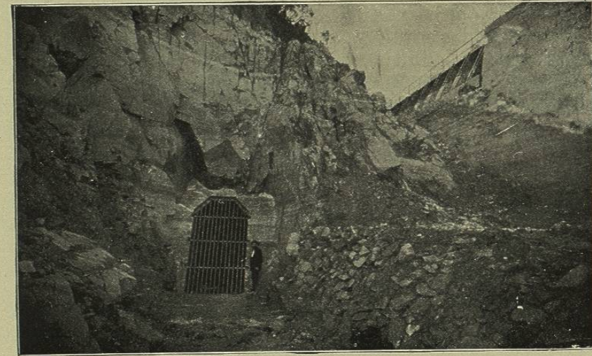
FIG. 163.—SWEETWATER DAM, SHOWING HEAD OF OUTLET TUNNEL AND SPILLWAY.
