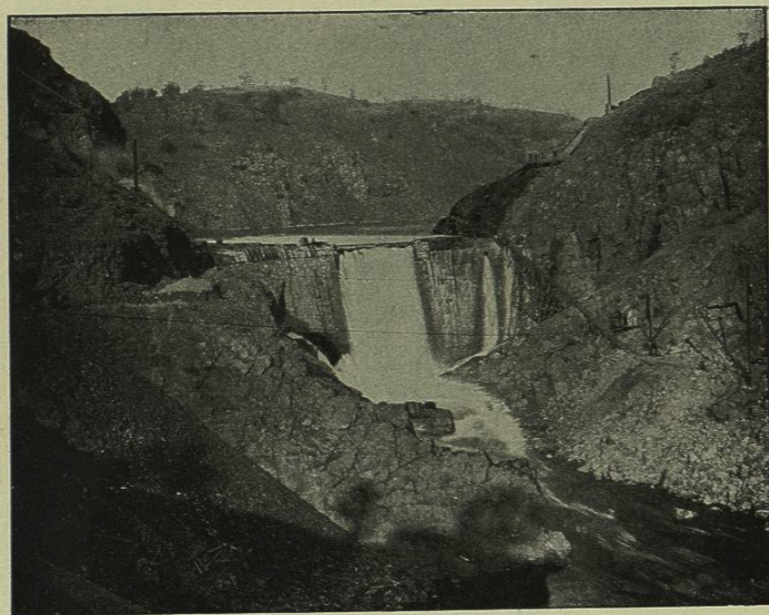
FIG. 182.—LA GRANGE DAM, CALIFORNIA.
