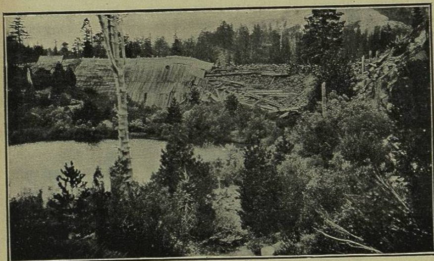
FIG. 347.—GENERAL VIEW OF THE TIMBER SKIN ON UP-STREAM SIDE OF THE ENGLISH LAKE DAM. NOW IN RUIN.
