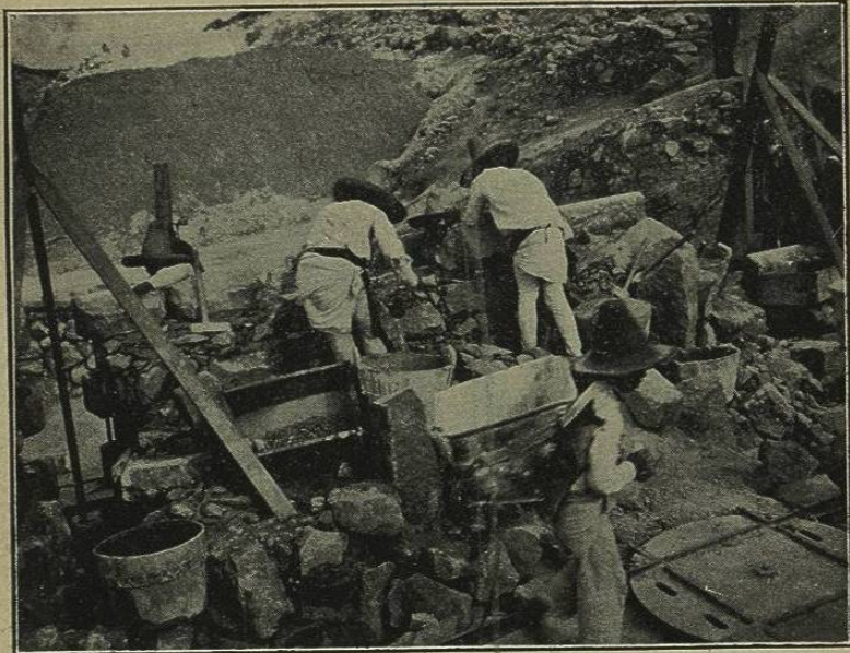
FIG. 374.—MASONS AT WORK ON THE SAN JOSÉ DAM, MEXICO.
