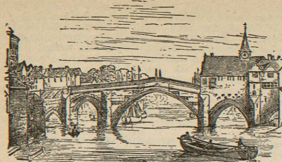
FIG. 115.—Old Bridge at York.
