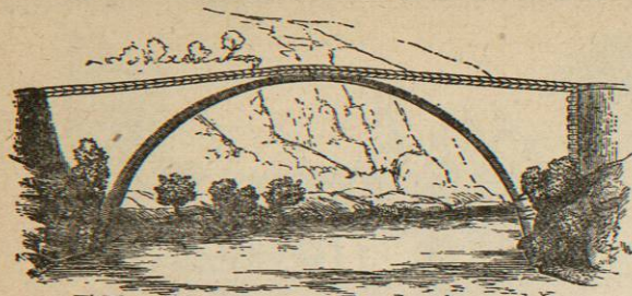
FIG. 112.—Bridge of Brioude.
