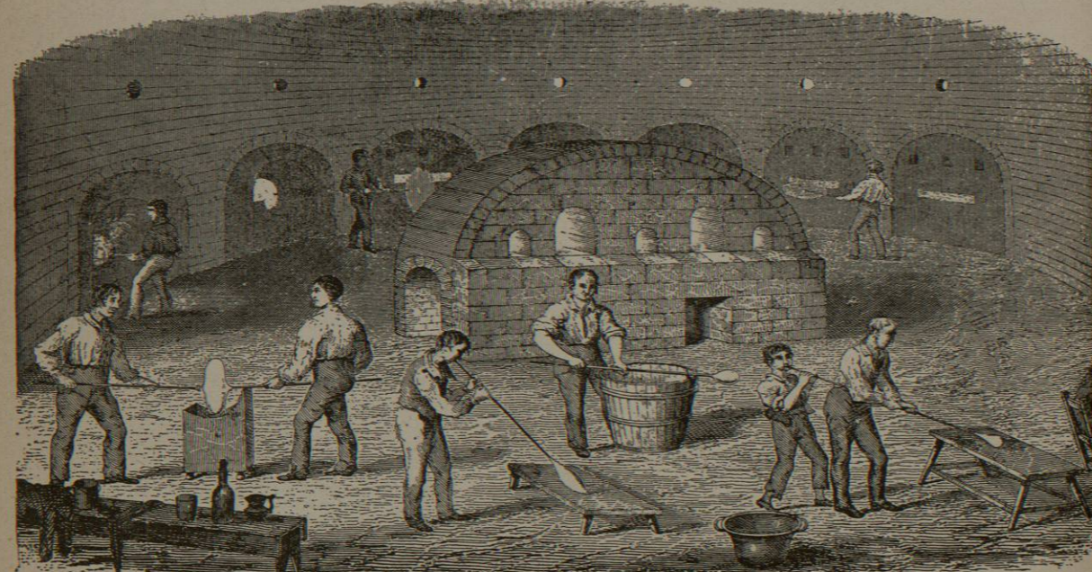
Fig. 2. INTERIOR OF A CROWN-GLASS HOUSE.
