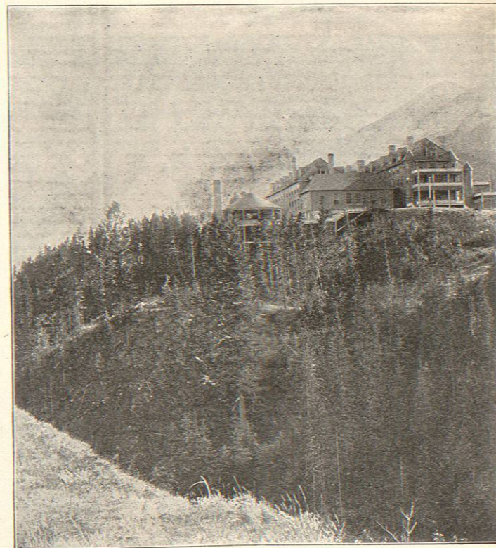
FIG. 474.—View of Hotel at Banff.
