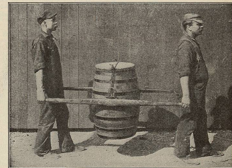
FIG. 3951.—Night-Soil Barrel, Used in Connection with Odorless Excavation Apparatus. (From Chapin's "Municipal Sanitation.")
