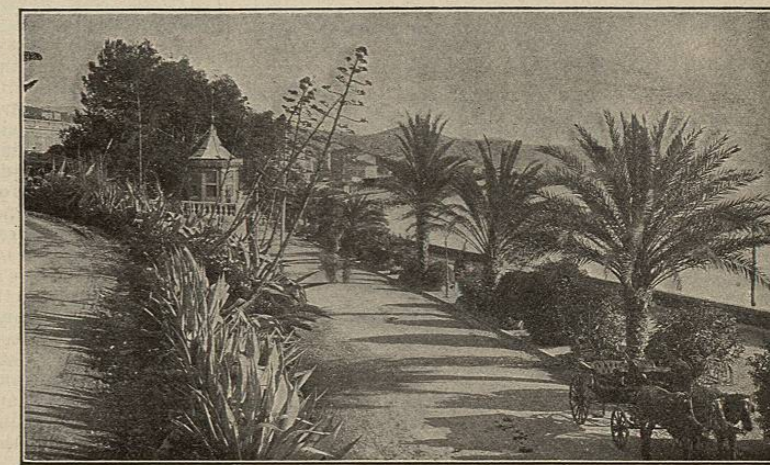
FIG. 4142.—Shore Drive and Promenade at San Remo.
