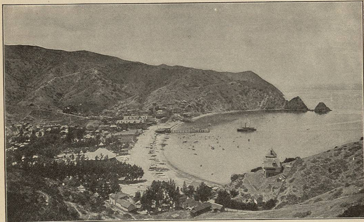
FIG. 4144.—Avalon in the Island of Santa Catalina, California.
