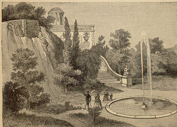
Construction of a Fountain.
