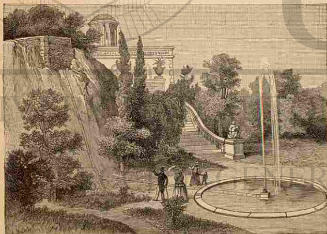
Construction of a Fountain.
