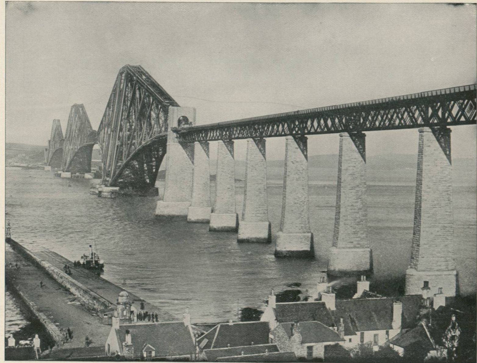
FORTH BRIDGE, SCOTLAND.—This bridge, crossing the Firth of Forth, is pronounced the largest structure in the world, and is the most striking feat yet achieved in bridge-building. It is 8296 feet long, 354 feet high, and cost $12,500,000. It was begun in 1883, and completed in 1890. It is built on the cantilever and central girder system, the principle of which is that of "stable equilibrium," its own weight helping to balance it more firmly in position. Each of the main spans is 1700 feet long, and the deepest foundations are 88 feet. The weight of the metal in the bridge is 50,000 tons.
