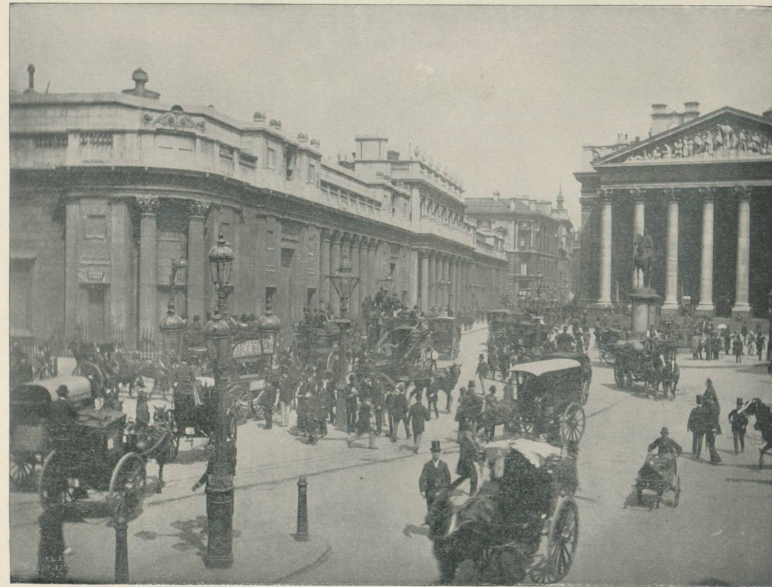
THE BANK OF ENGLAND, LONDON, ENGLAND.—The irregular, isolated, one-story building, covering an area of four acres, and located in the central part of London, is the largest and most powerful institution in the world. It is the only bank in London which has the power to issue paper money; its average daily business is over $10,000,000. It employs 900 people, and usually carries in its vaults from $75,000,000 to $100,000,000, while there are from 100 to 125,000,000 dollars of the bank's notes in circulation. On the right is the Stock Exchange, giving 1000 stock brokers daily employment.
