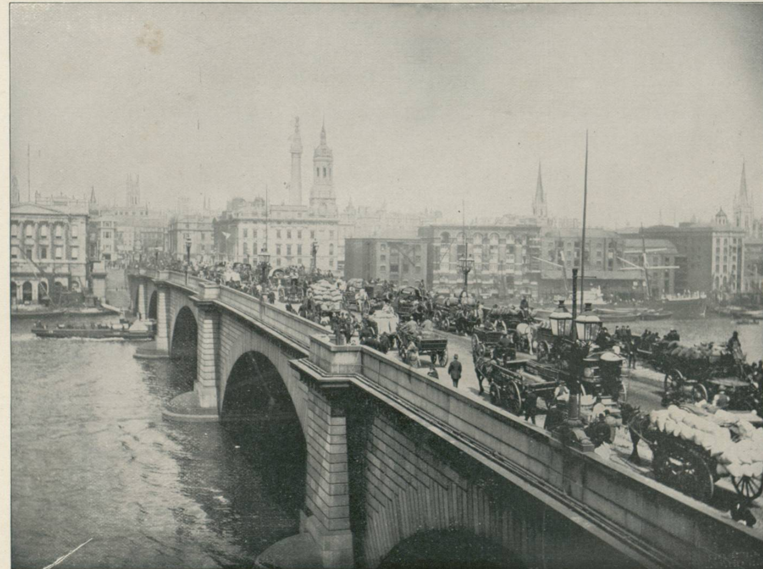
LONDON BRIDGE, LONDON, ENGLAND.—Centuries ago the Saxons and Romans erected various wooden bridges over the Thames, on the site of the present London Bridge; but they were all carried away by floods, or destroyed by fire. This bridge was begun in 1825 and completed in 1831 at a cost of $10,000,000. The bridge, 928 feet long and 54 feet wide, is borne by five granite arches, that in the centre having a span of 152 feet. The lamp-posts on the bridge are cast of the metal of French cannons captured in the Peninsular War. About 15,000 vehicles and 100,000 pedestrians cross the bridge daily.
