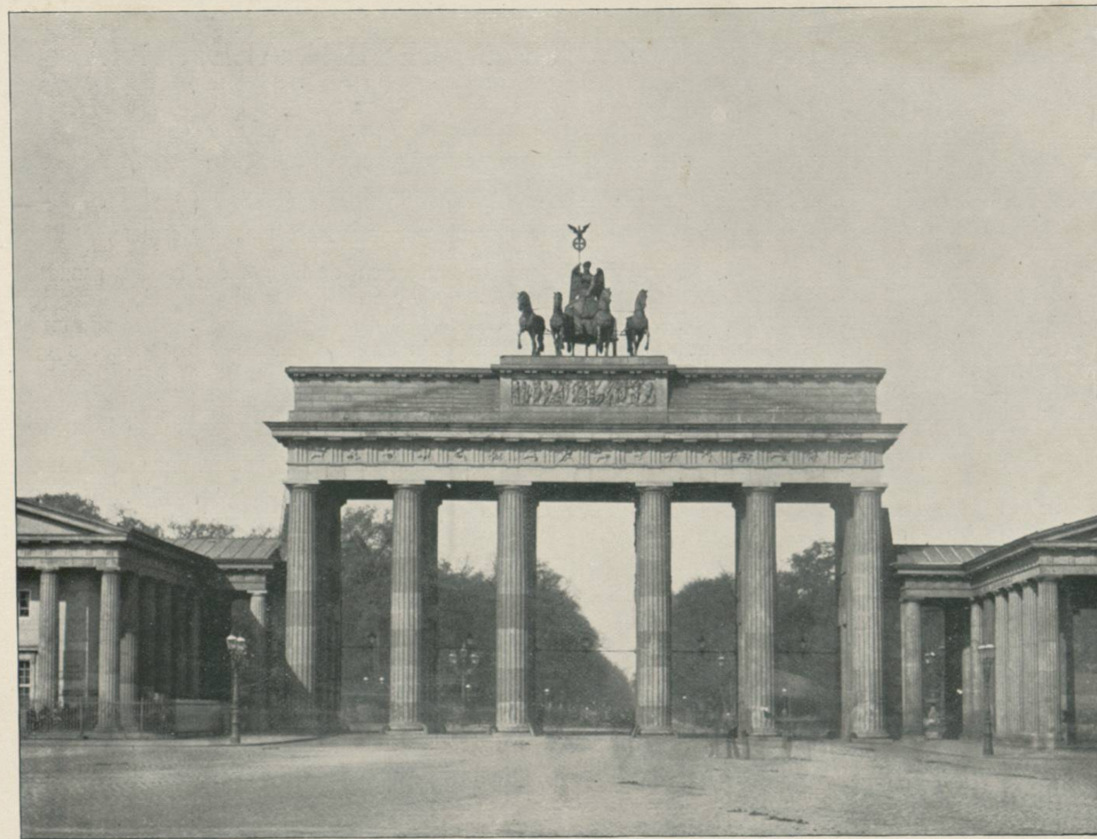
THE BRANDENBURG GATE, BERLIN, GERMANY.—The Brandenburg Gate, forming the entrance to Berlin, from the Thiergarten, was erected in 1793 in imitation of the Propylæa at Athens. It is 85 feet high and 205 feet wide, and has five different passages, separated by massive Doric columns. It is at the one end of "Unter den Linden," and its middle passage is reserved for royal carriages only. The material is sandstone, and it is surmounted by a Quadriga of Victory from copper, taken to Paris by Napoleon in 1807, but restored in 1814. On the side are two wings resembling Grecian Temples, one of which is a pneumatic post-office and the other a guard-house. Both combine in their construction, strength, elegance and beauty.
