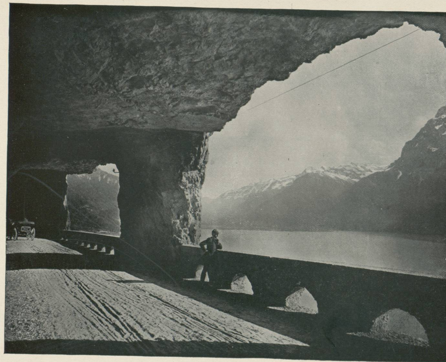
AXENSTRASSE, SWITZERLAND.—This famous road extends nine miles along the Lake of Uri, from Brunnen to Fluelen, and is noted for the remarkable boldness displayed in its construction. It is to a great extent hewn out of solid rock, cut like a shelf into the side of the mountain, with occasional pillars to hold the thousands of tons of rock above, and a strong balustrade to guard travellers from tumbling over the abrupt precipice into the lake many feet below. It is the great highway leading from Switzerland to Italy, and is regarded as one of the most picturesque roads in the world.
