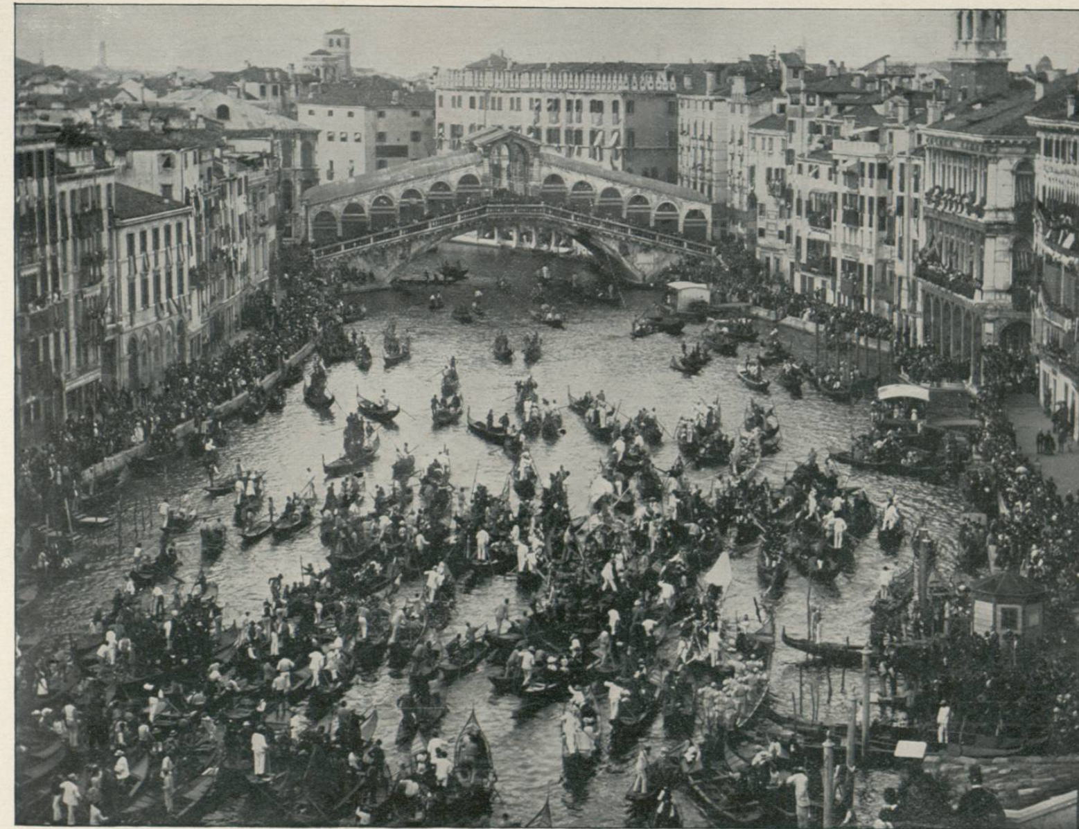
THE RIALTO, VENICE, ITALY.—This famous bridge, one hundred and fifty-eight feet long and forty-six feet wide, rests on twelve hundred posts. It was erected from 1588 to 1591. Its sides are lined with little shops, extending from a fish-market at one end, past jewelry-shops in the centre of the structure, down to a fruit-market at the other side. It always presents a busy appearance, and is considered a marvel of engineering skill, and one of the finest bridges in the world. The picture represents the annual parade on the Grand Canal, with the Rialto in the background, which is always the rallying centre on such occasions.
