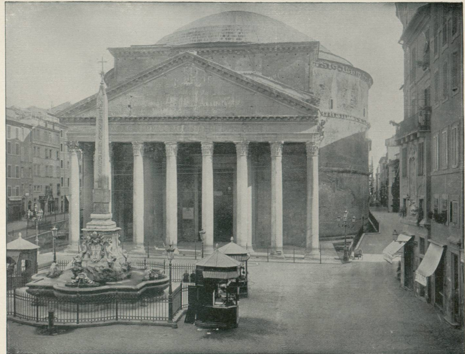
PANTHEON, ROME, ITALY.—This is the only ancient edifice at Rome which is still in perfect preservation, as regards the walls and vaulting. The original statues and architectural decorations have long since been replaced by modern and inferior works, but the huge circular structure with its vast colonnade still presents a strikingly imposing appearance. The walls are twenty feet in thickness and were originally covered with marble and stucco. The height and diameter of the dome are each one hundred and forty feet. The opening of the dome at the top is thirty feet in diameter, and through this aperture the ancients supposed the gods to descend. The building is supposed to have been constructed in the first century B. C.
