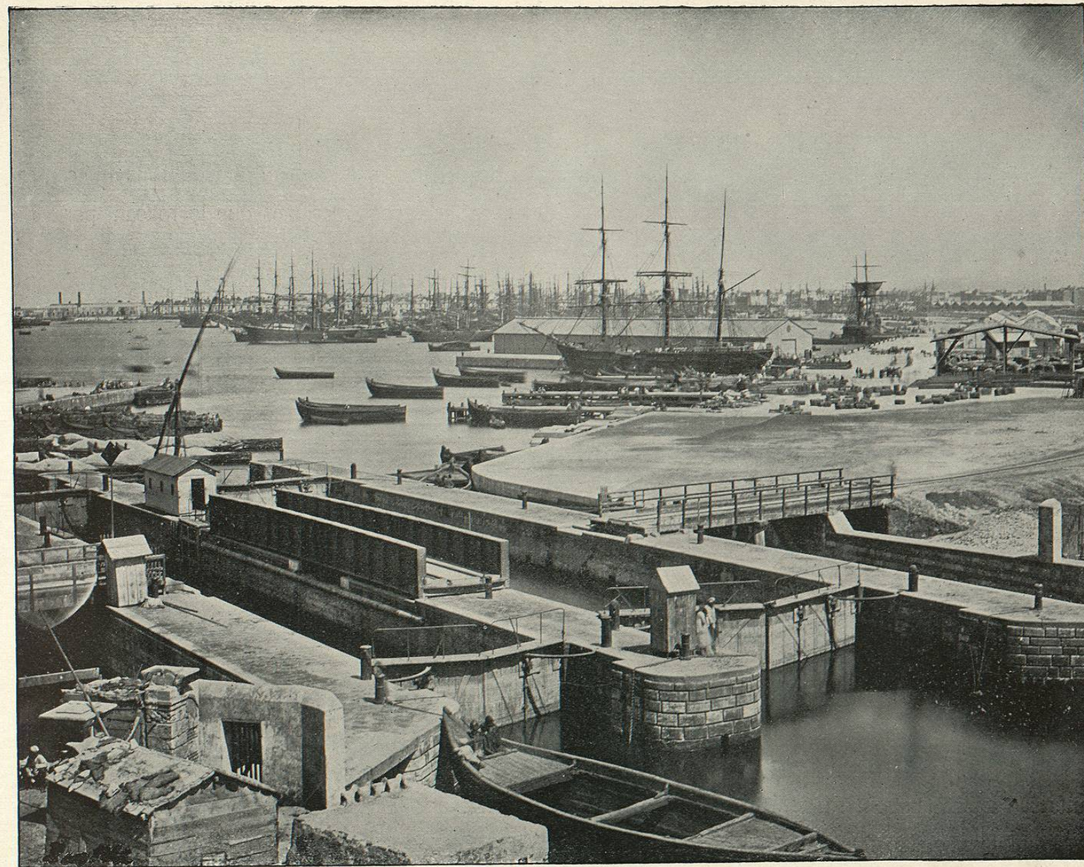
HARBOR, ALEXANDRIA, EGYPT.—The perfectly flat coast of Egypt, and even Alexandria itself, are not visible to the steam-boat passenger until very shortly before the vessel enters the harbor. The latter consists of an outer breakwater, forming an obtuse angle nearly two miles in length. A second pier, nearly a mile in length, protects an inner harbor covering nearly five hundred acres of water, twenty-seven feet deep. No fewer than thirty thousand artificial blocks, weighing twenty tons each, and two million tons of natural blocks of stone were used in the construction of these magnificent harbor works.
