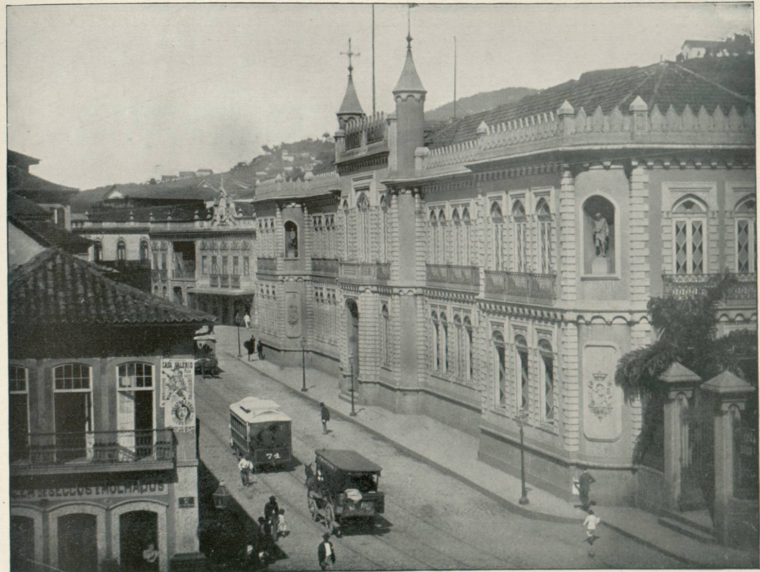
STREET SCENE, RIO DE JANEIRO, SOUTH AMERICA.—The streets of Rio de Janeiro do not impress the traveller favorably. They are excessively narrow and the buildings by no means handsome. In the southern division of the city, the streets, one of which is shown in the photograph, are much more open and attractive. This is the fashionable district, and contains many delightful residences. The city itself, during business hours, is full of activity. Immense numbers of negroes crowd continually up and down with heavy bags and bales. The government of Brazil has been making great efforts to improve the condition of the streets and good progress is being made.
