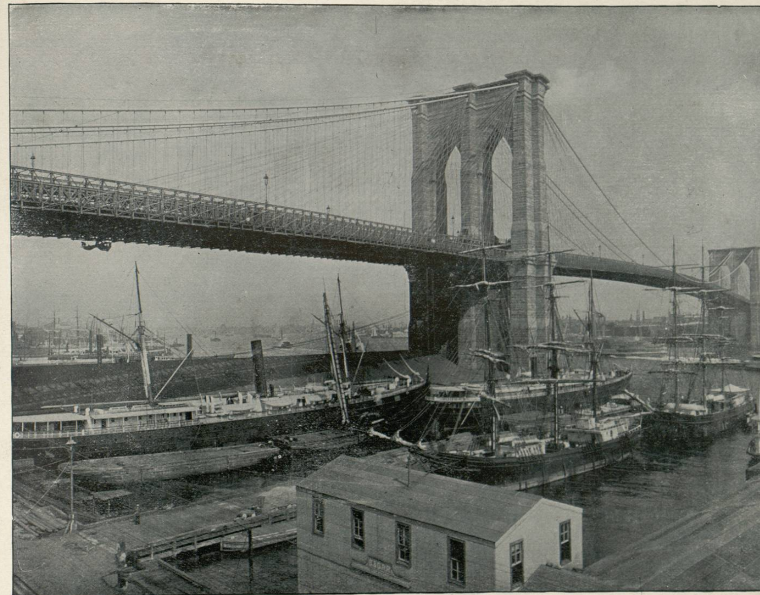
BROOKLYN BRIDGE, NEW YORK CITY, N. Y.—This bridge, connecting New York with Brooklyn, is by far the largest suspension bridge yet constructed. The work was commenced in 1870, and opened for traffic on May 24, 1883. The central span, from tower to tower, measures fifteen hundred and ninety-five and one-half feet. In the centre is a foot-way, fifteen and one-half feet wide, and raised twelve feet above the other passages, affording an open view on both sides. There are tracks on each side for cable cars, worked by a stationary engine on the Brooklyn side, and on the outside are wagon-ways. The entire cost was $15,500,000.
