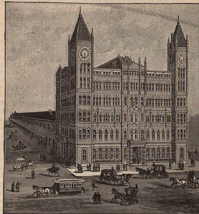
Estacion del Ferrocarril Lake Shore & Michigan Southern—Chicago.
