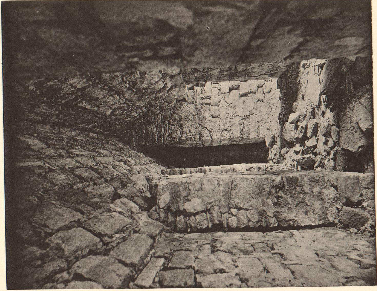
2. YASCHILAN: INTERIOR STRUCTURE, 40.
