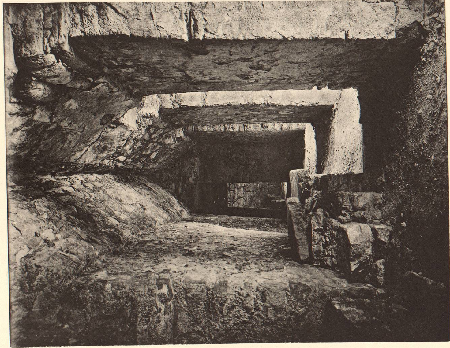
1. YASCHILAN: INTERIOR STRUCTURE, 19.
