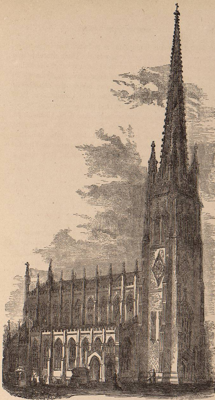
TRINITY CHURCH—Broadway opposite, Wall Street; 80 x 192 feet; 284 feet high.
