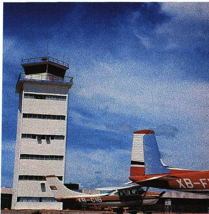
Fig.9.1 Torre de control
